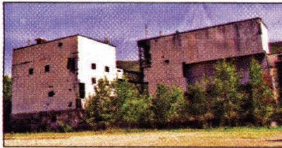
Demolition of this derelict structure in the mill complex is scheduled to begin soon.
