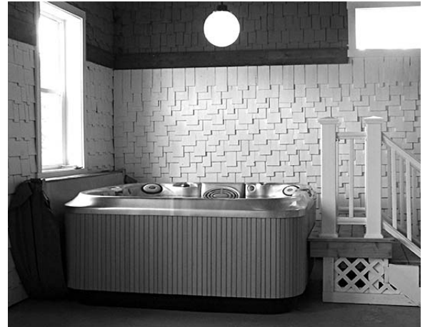
New stairs and railing for hot tub
