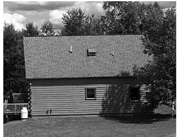
New staining on cabin
