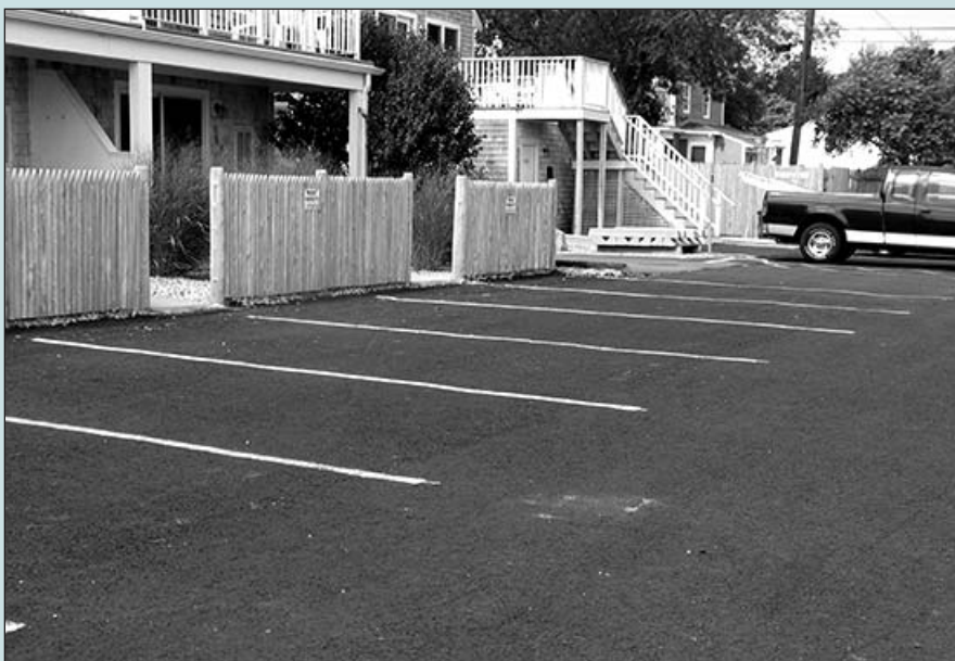
Initial Coating of Parking Lot
