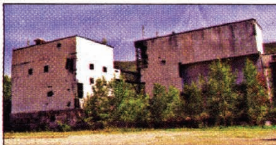
Demolition of this derelict structure in the mill complex is scheduled to begin soon.
